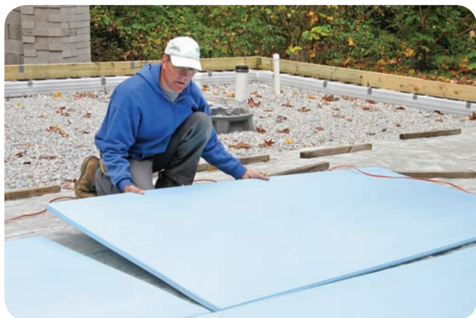
▲ Polystyrene is an insulator: it helps to prevent heat loss. So it is used under floors, and in fast-food cartons.
