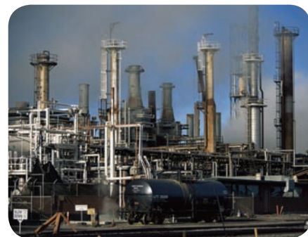
▲ A petroleum refinery. It produces petrol and many other useful substances, with the help of fractional distillation.
