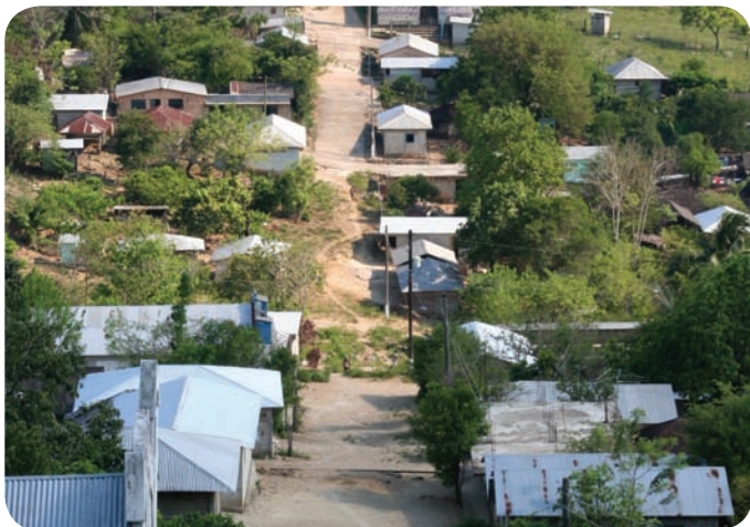
▲ Roofs of galvanised iron in a Mexican village. It is usually called corrugated iron .
